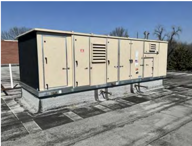
9 - ROOF MOUNTED AIR HANDLING UNIT
