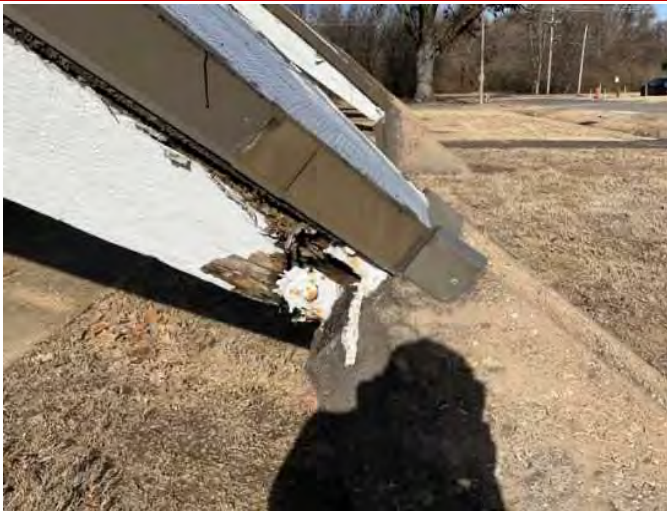
7 - WOOD ROT AT ROOF STRUCTURE (GYMNASIUM)
