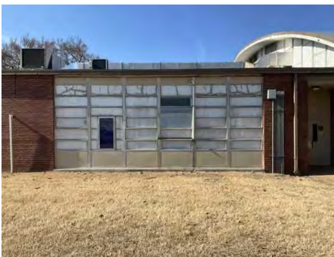
5 - SINGLE PANE STEEL FRAME WINDOWS
