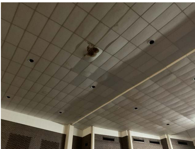
29 - ROOF LEAK DAMAGE
