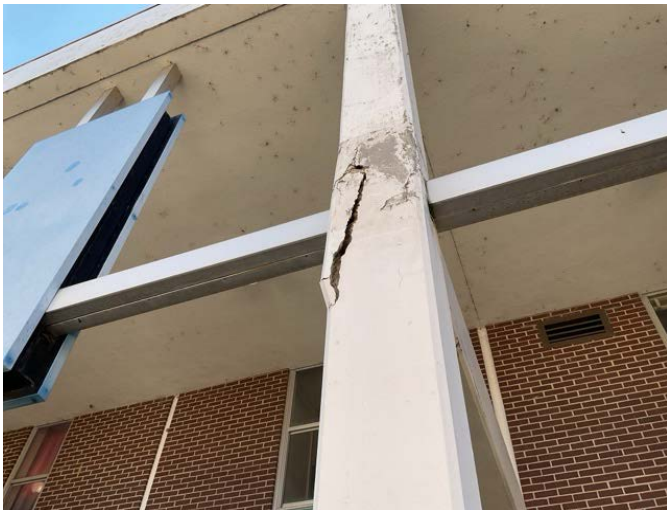
21 - STRUCTURAL DETERIORATION
