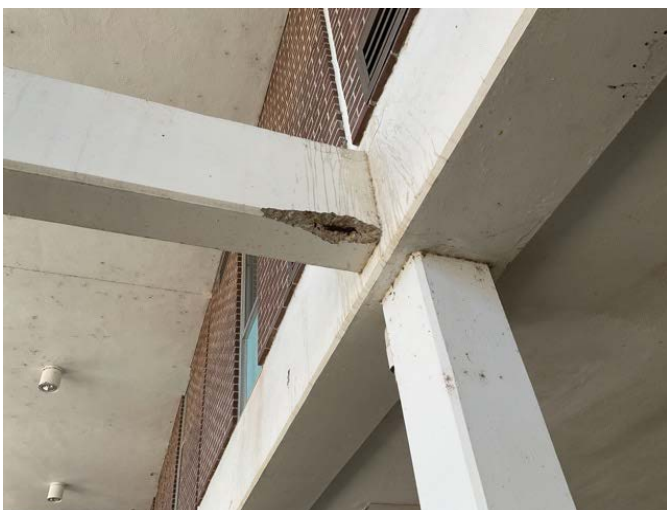
23 - STRUCTURAL DETERIORATION
