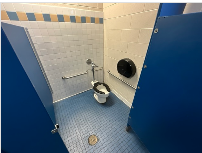
TOILET STALL OVERVIEW
