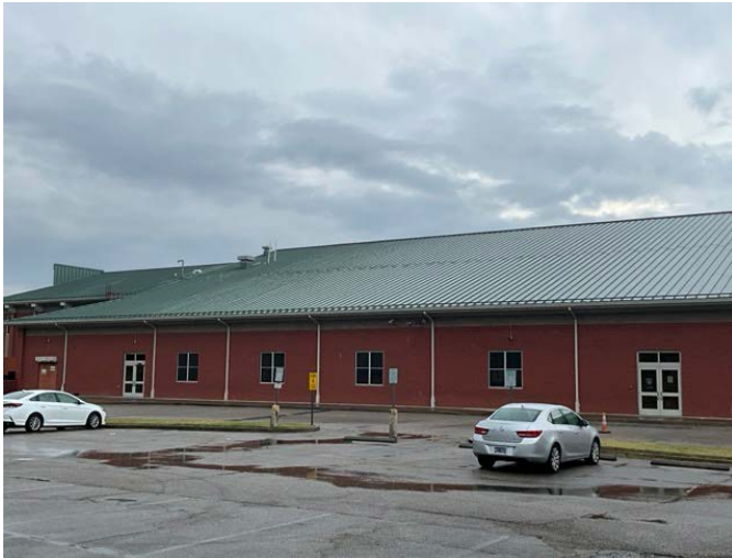
7 - PRIMARY ROOF OVERVIEW
