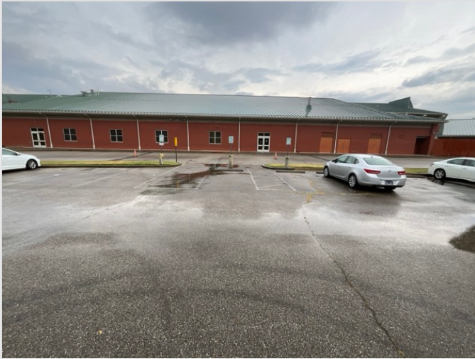
OVERVIEW OF ACCESSIBLE PARKING AREA
