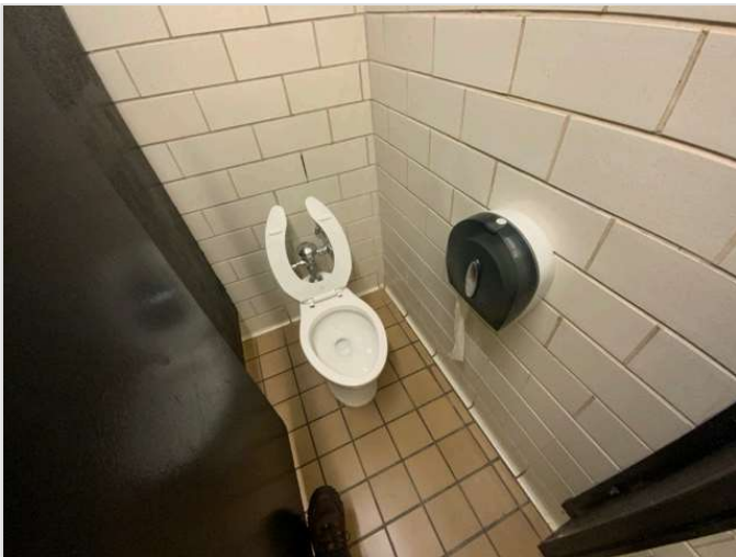
TOILET STALL OVERVIEW
