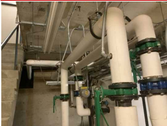
19 - DUAL TEMPERATURE PIPING
