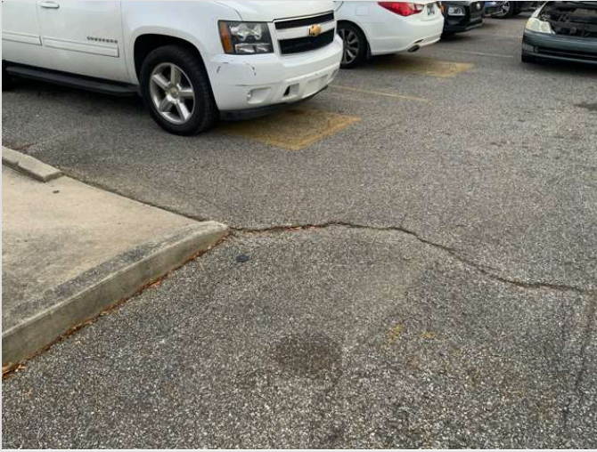
OVERVIEW OF ACCESSIBLE PARKING AREA
