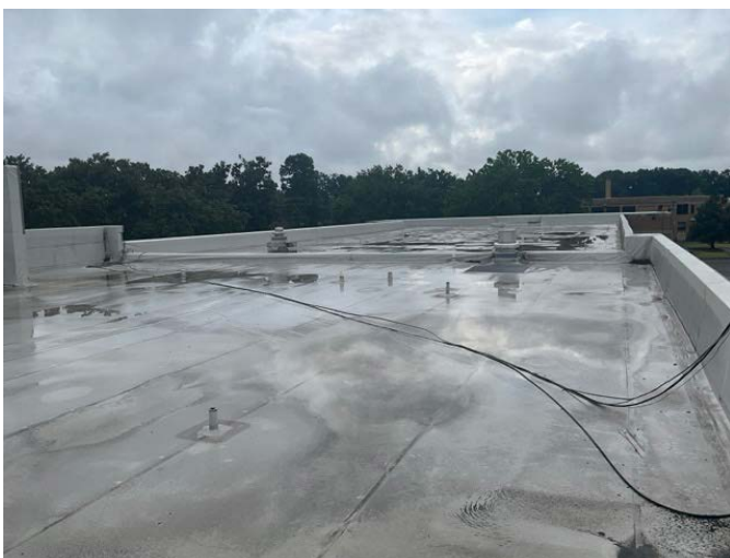
5 - PRIMARY ROOF OVERVIEW
