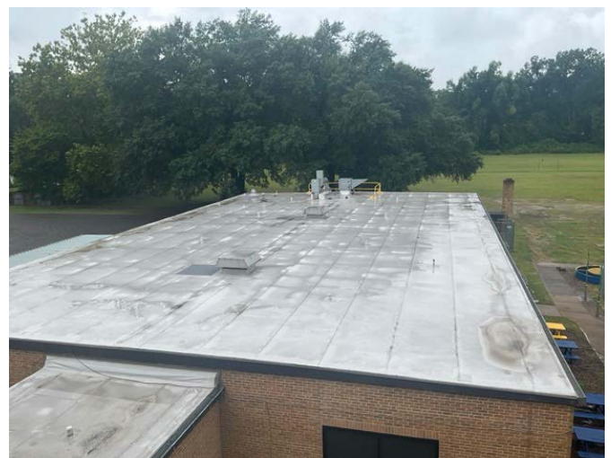
6 - SECONDARY ROOF OVERVIEW
