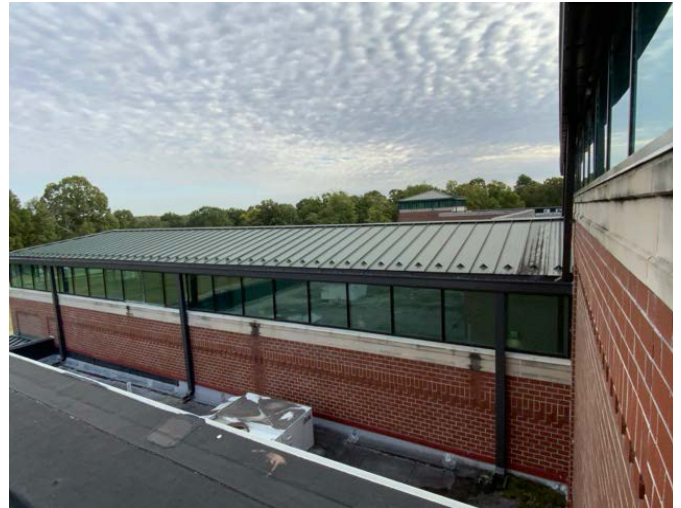
8 - SECONDARY ROOF OVERVIEW
