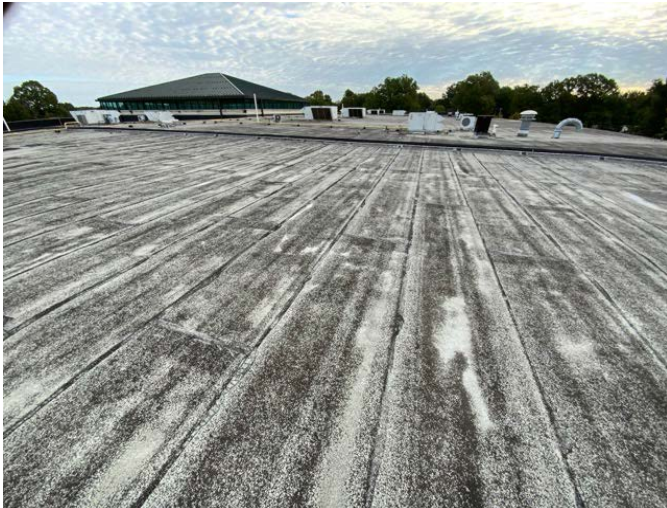
7 - PRIMARY ROOF OVERVIEW
