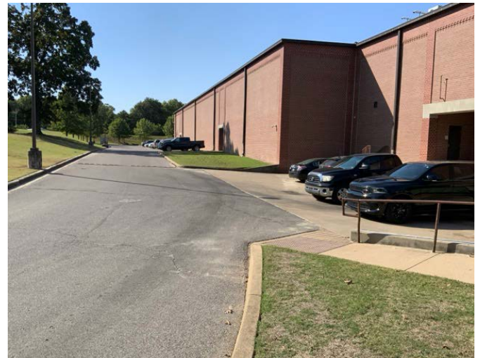
34 - SECONDARY PARKING AREA
