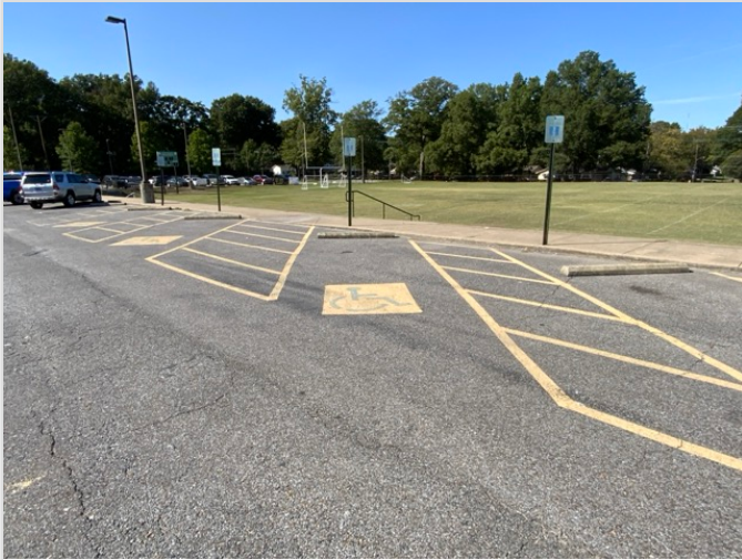
OVERVIEW OF ACCESSIBLE PARKING AREA
