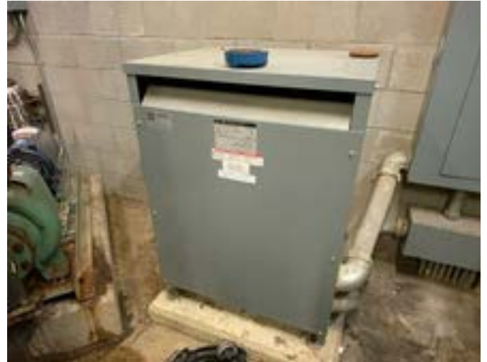
38 - SECONDARY TRANSFORMER
