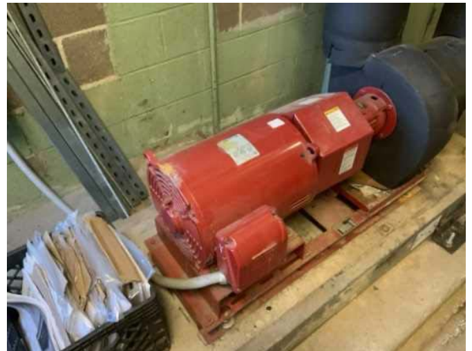
22 - HEATING WATER DISTRIBUTION PUMP
