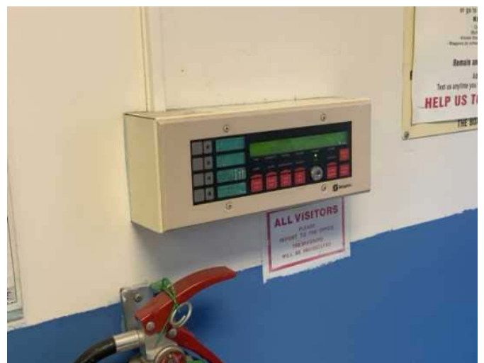
30 - FIRE ALARM SYSTEM ANNUNCIATOR
