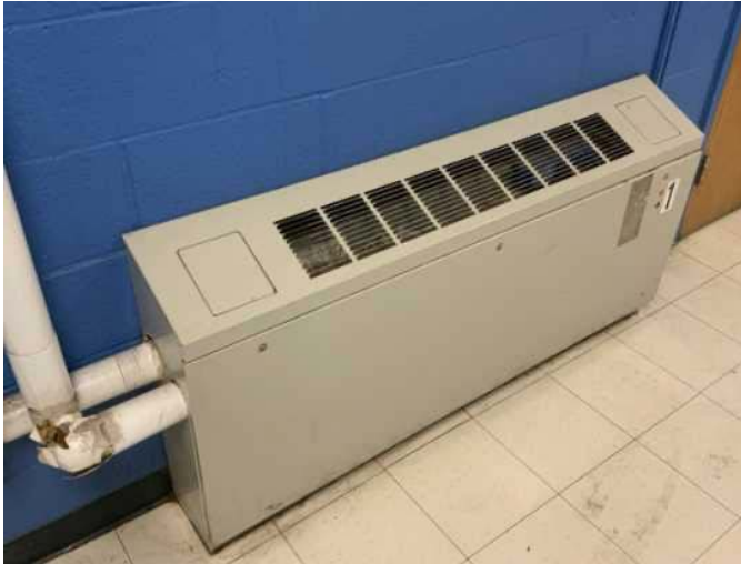
25 - TYPICAL FAN COIL UNIT
