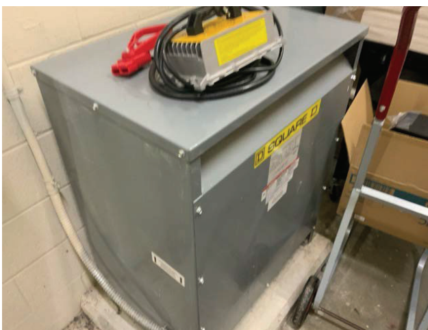
23 - SECONDARY TRANSFORMER
