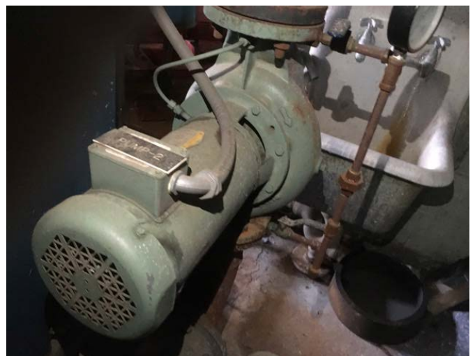
24 - PUMP, HVAC HEATING WATER
