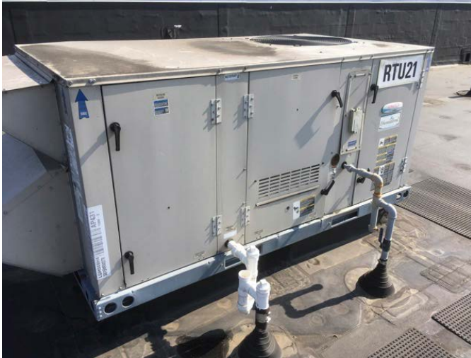
25 - PACKAGED UNIT, RTU
