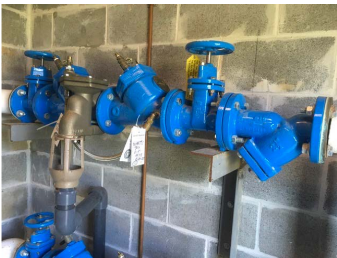
17 - BACKFLOW PREVENTER, DOMESTIC WATER
