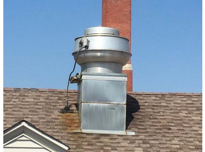
26 - EXHAUST FAN, CENTRIFUGAL
