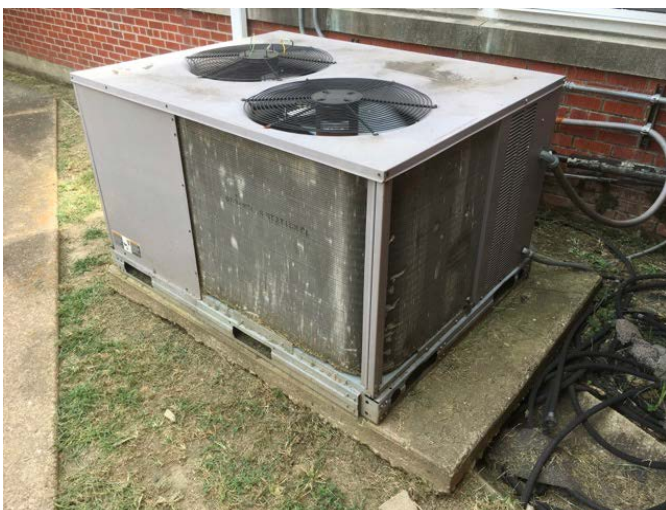
23 - SPLIT SYSTEM, CONDENSING UNIT
