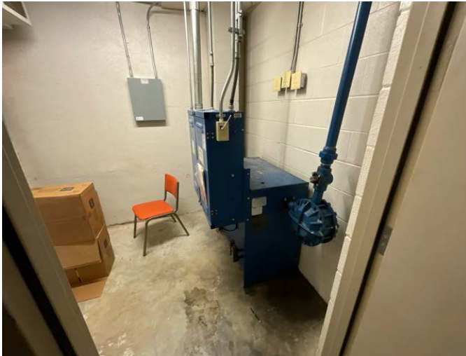
25 - ELEVATOR MACHINERY
