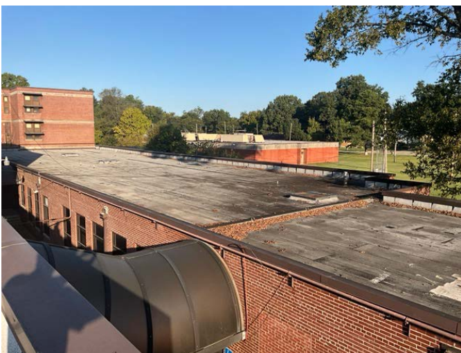
5 - PRIMARY ROOF OVERVIEW
