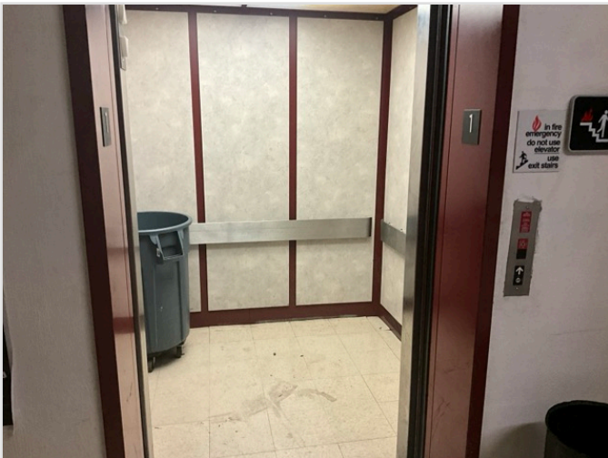
LOBBY LOOKING AT CABS (WITH DOORS OPEN)
