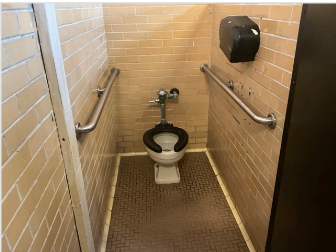
TOILET STALL OVERVIEW
