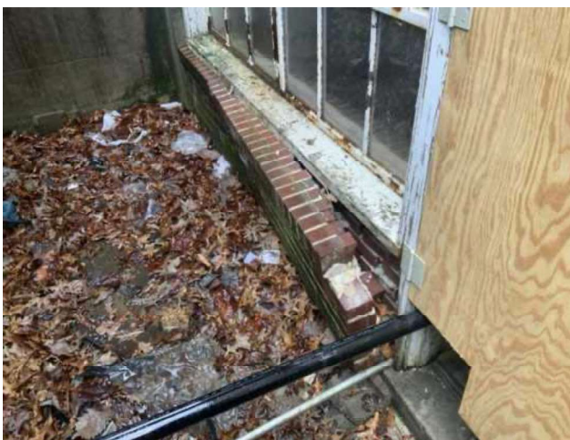
17 - DAMAGED BRICK VENEER
