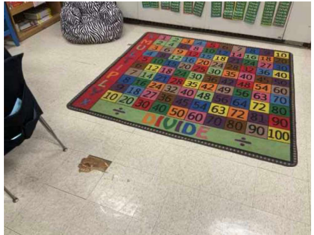
28 - SUB-FLOOR FAILURE IN CLASSROOMS
