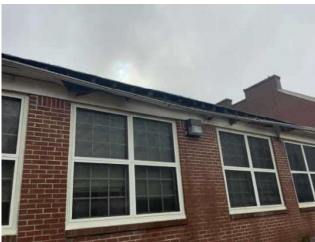
11 - DAMAGED SOFFIT AND FASCIA
