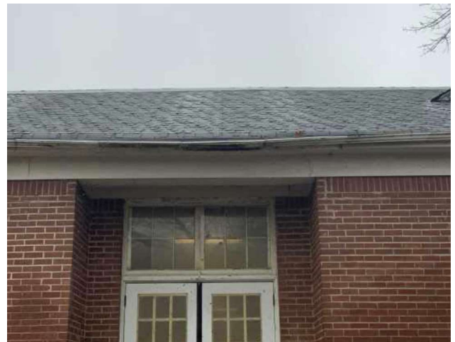
16 - DAMAGED SOFFIT AND FASCIA
