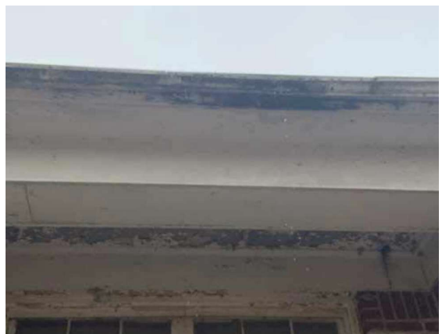
12 - DAMAGED SOFFIT AND FASCIA
