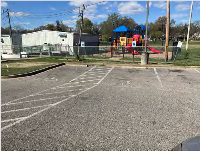
OVERVIEW OF ACCESSIBLE PARKING AREA
