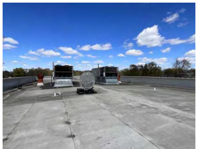
6 - PRIMARY ROOF OVERVIEW
