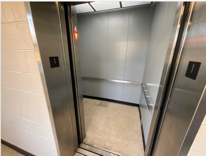
LOBBY LOOKING AT CABS
