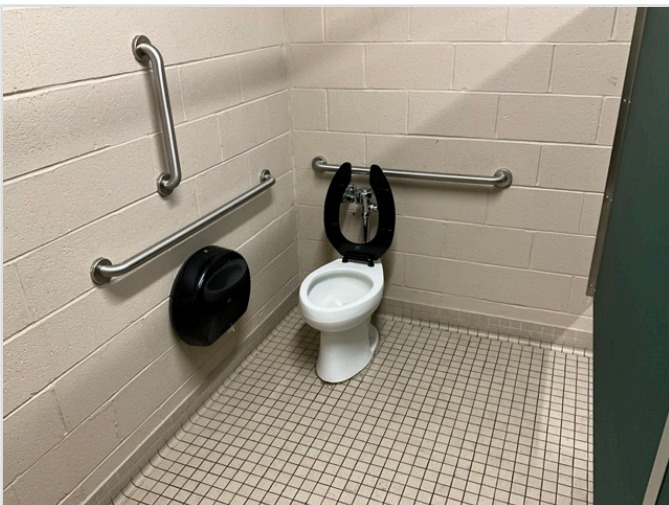
TOILET STALL OVERVIEW
