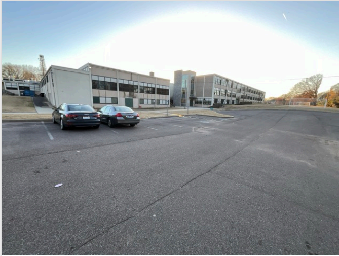
OVERVIEW OF ACCESSIBLE PARKING AREA
