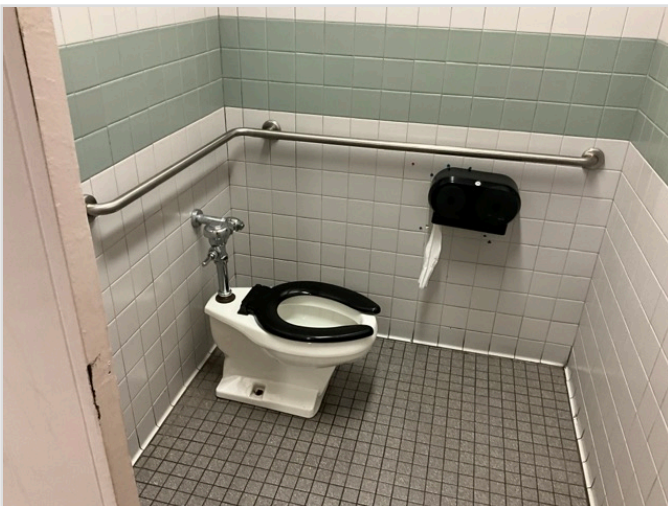
TOILET STALL OVERVIEW
