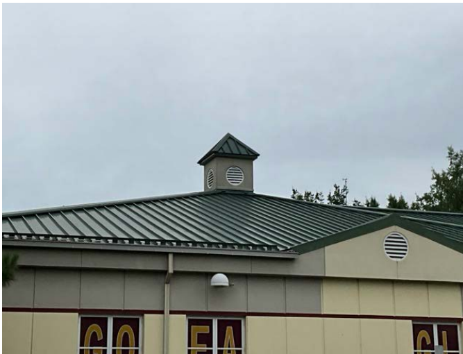
9 - PRIMARY ROOF OVERVIEW
