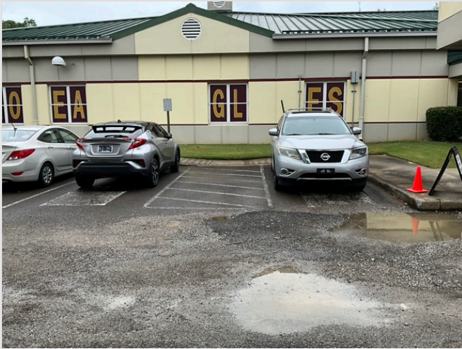
OVERVIEW OF ACCESSIBLE PARKING AREA
