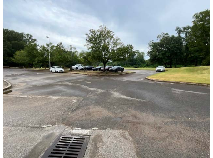
26 - SECONDARY PARKING AREA
