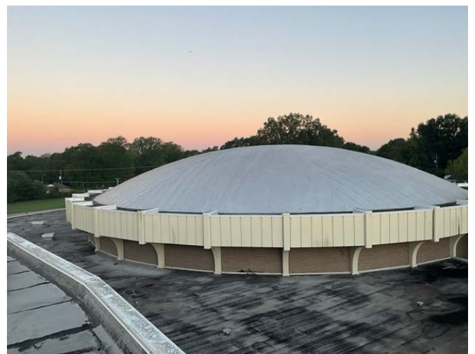
6 - SECONDARY ROOF OVERVIEW
