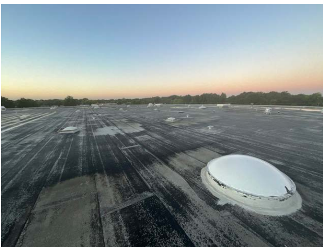
5 - PRIMARY ROOF OVERVIEW
