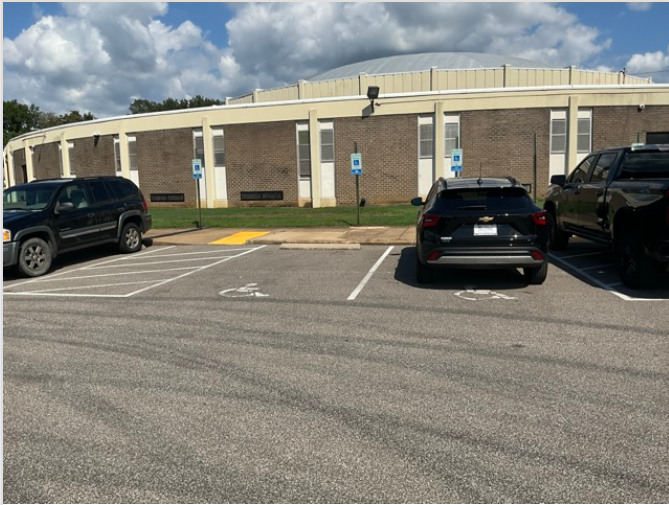
OVERVIEW OF ACCESSIBLE PARKING AREA
