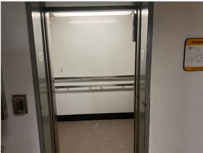
LOBBY LOOKING AT CABS (WITH DOORS OPEN)
