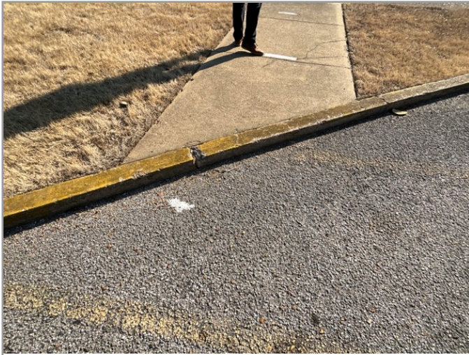
ACCESSIBLE ROUTE TO PLAYGROUND
