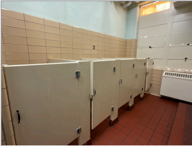
TOILET STALL OVERVIEW
