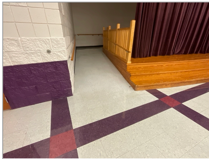
ACCESSIBLE INTERIOR RAMP
