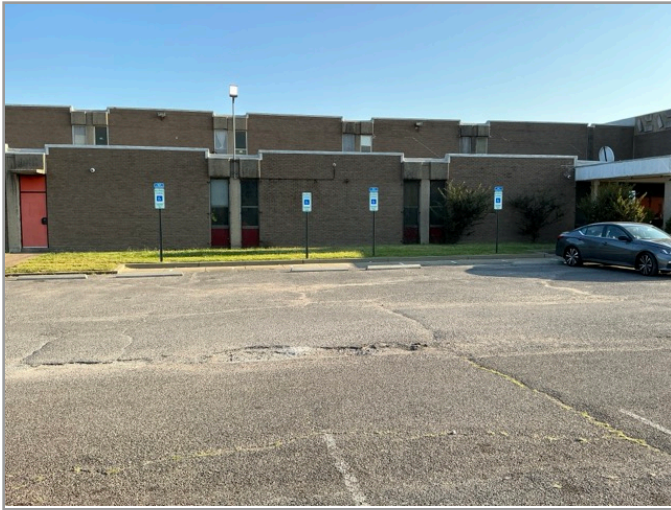
OVERVIEW OF ACCESSIBLE PARKING AREA
