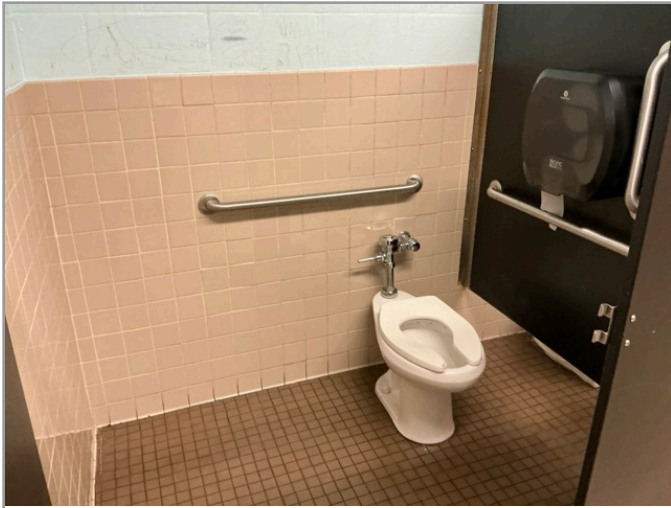
TOILET STALL OVERVIEW
