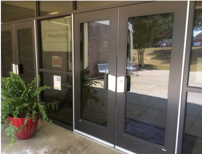
7 - EXTERIOR DOOR, ALUMINUM AND GLAZED
