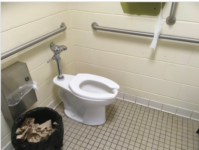
TOILET STALL OVERVIEW
