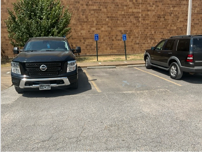
OVERVIEW OF ACCESSIBLE PARKING AREA
