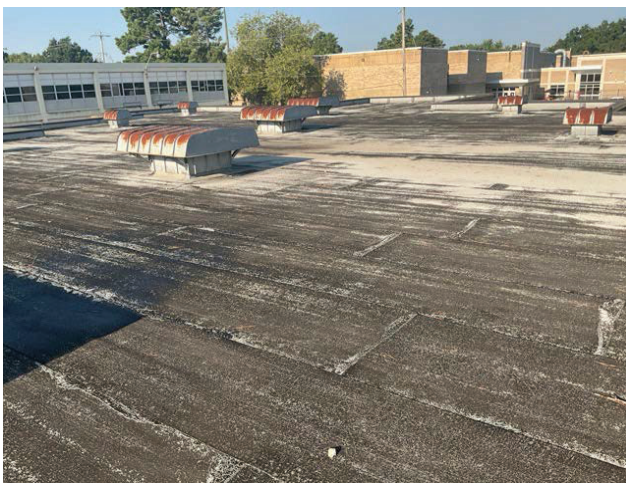
5 - PRIMARY ROOF OVERVIEW
