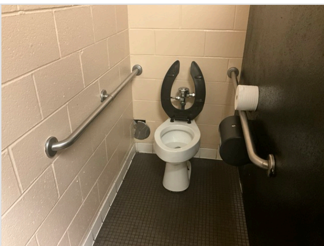
TOILET STALL OVERVIEW
