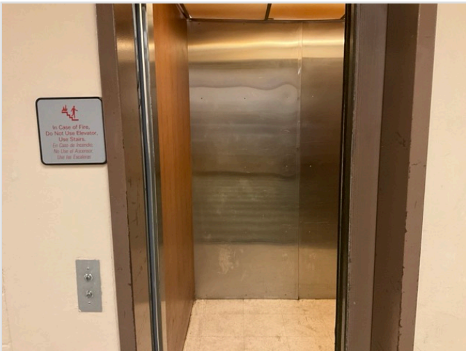
LOBBY LOOKING AT CABS (WITH DOORS OPEN)
