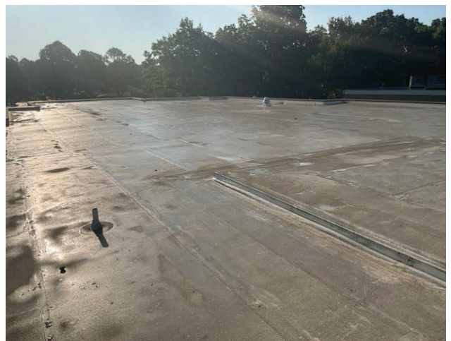
6 - SECONDARY ROOF OVERVIEW
