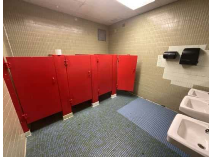
32 - RESTROOM (MAIN BUILDING)
