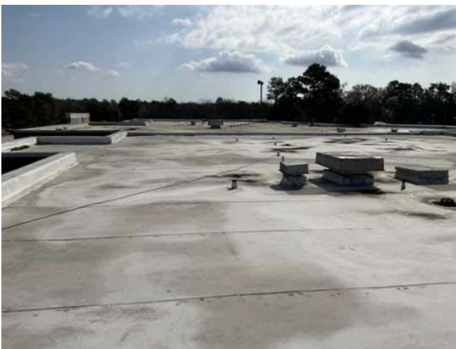
5 - MAIN BUILDING ROOF
