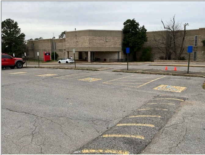
OVERVIEW OF ACCESSIBLE PARKING AREA
