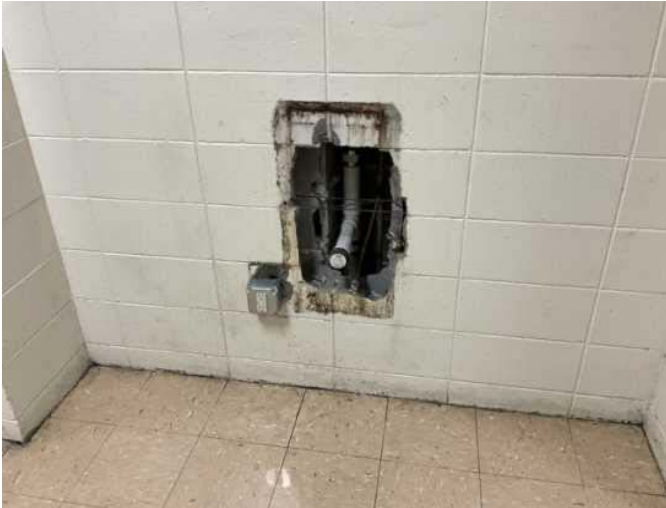
31 - ROUGH OPENING IN WALL
