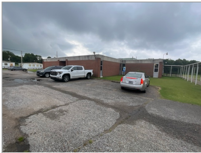
OVERVIEW OF ACCESSIBLE PARKING AREA
