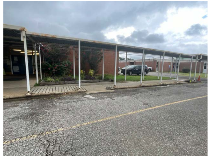
28 - SIDEWALKS AND LANDSCAPING
