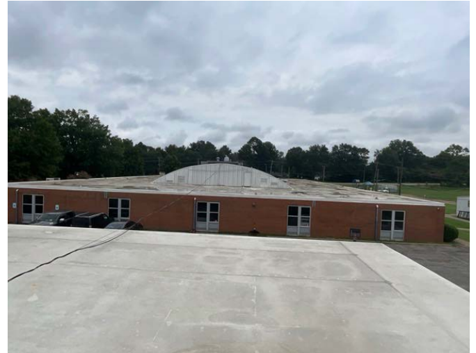
8 - SECONDARY ROOF OVERVIEW
