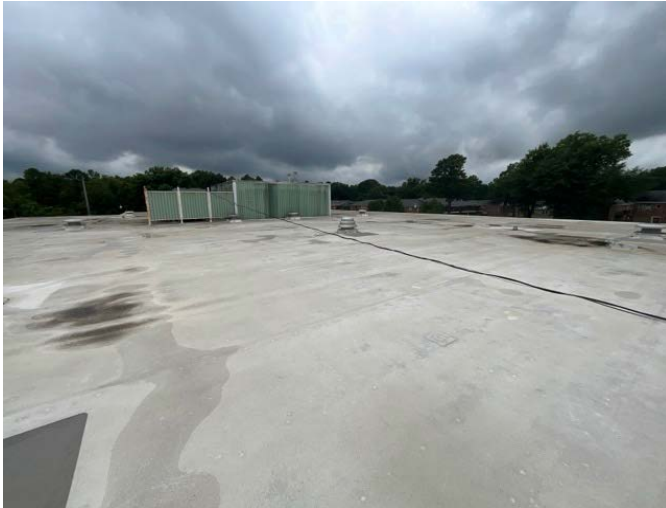
7 - PRIMARY ROOF OVERVIEW
