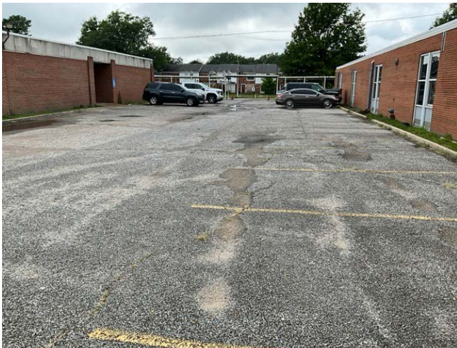
27 - SECONDARY PARKING AREA
