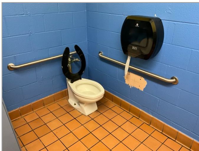
TOILET STALL OVERVIEW
