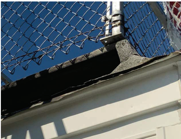
9 - MODIFIED BITUMEN ROOFING
