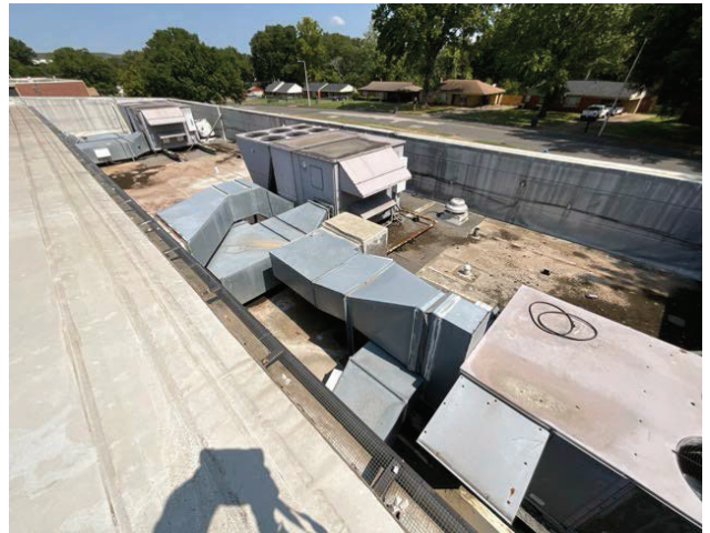
22 - ROOF OVERVIEW - AUDITORIUM
