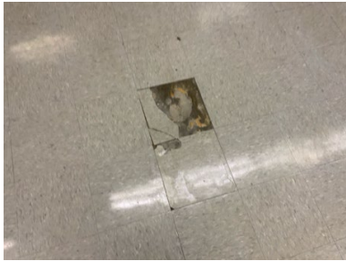
Some broken tiles - AssetCALC ID: 8205614
