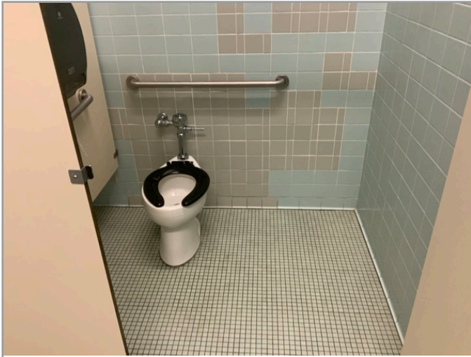
TOILET STALL OVERVIEW
