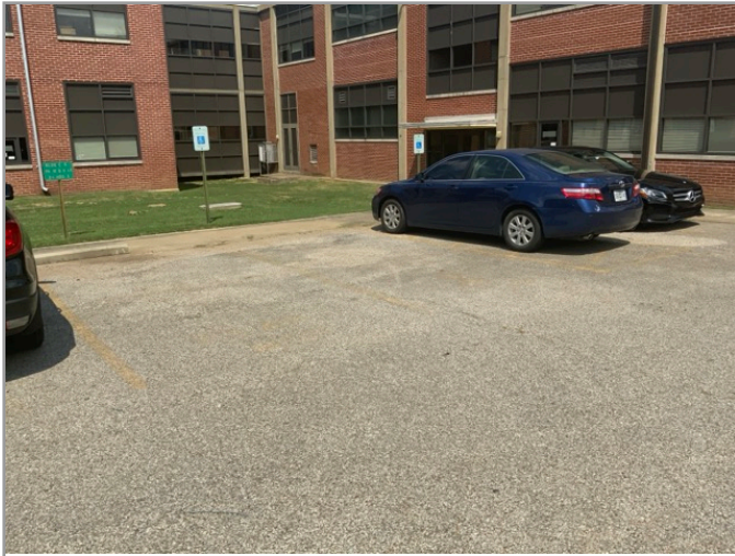
OVERVIEW OF ACCESSIBLE PARKING AREA
