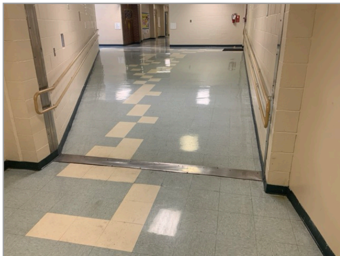
ACCESSIBLE INTERIOR RAMP
