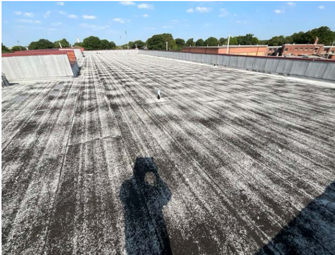
7 - ROOFING OVERVIEW - MODIFIED BITUMEN
