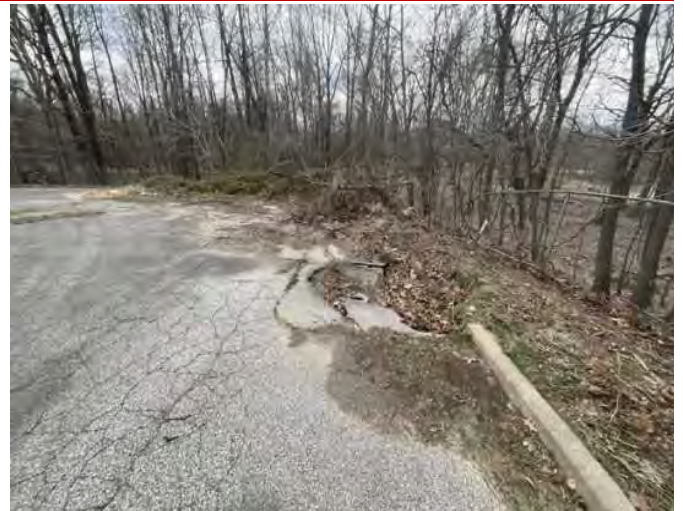
8 - PARKING LOT DETERIORATION
