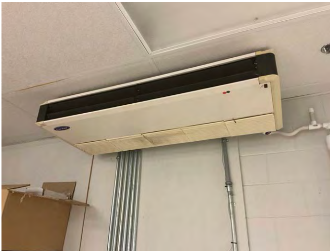
15 - SPLIT SYSTEM DUCTLESS
