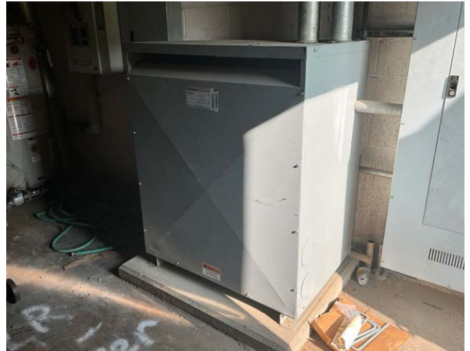
32 - STEP-DOWN TRANSFORMERS & PANELS
