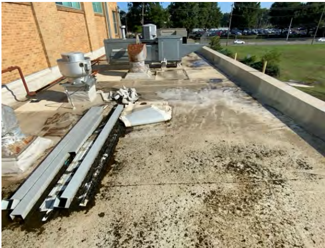
9 - SECONDARY ROOF OVERVIEW
