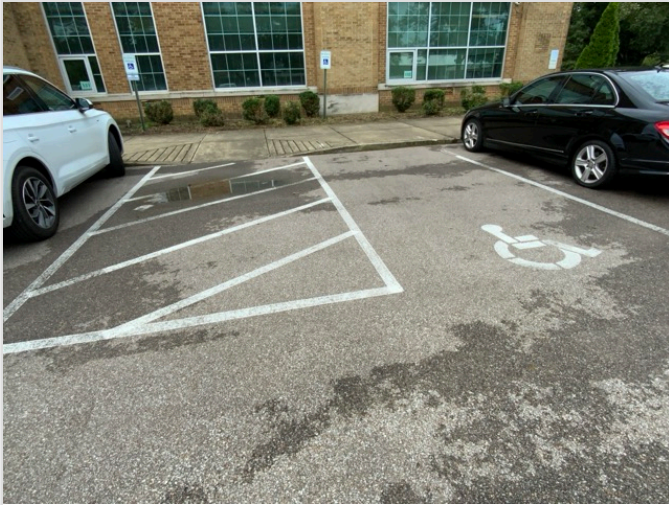
OVERVIEW OF ACCESSIBLE PARKING AREA
