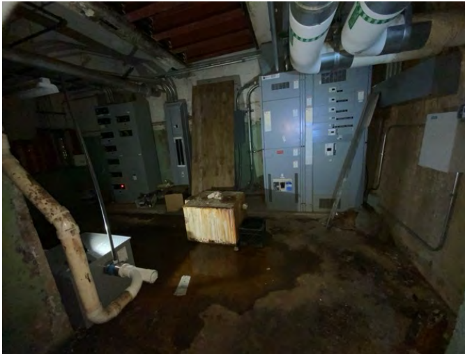
25 - MAIN ELECTRICAL ROOM
