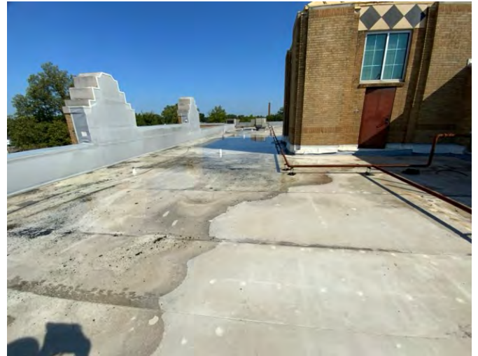
8 - PRIMARY ROOF OVERVIEW
