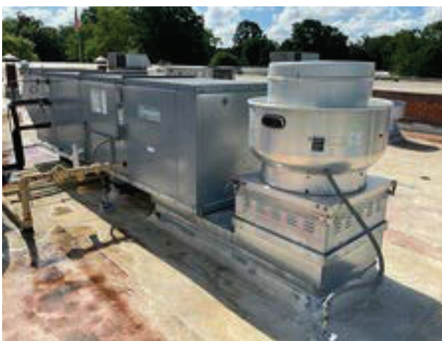
17 - MAKE-UP AIR AND EXHAUST
