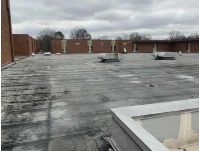
7 - MODIFIED BITUMEN ROOF
