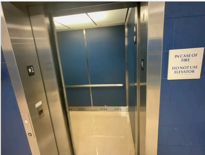
LOBBY LOOKING AT CABS
