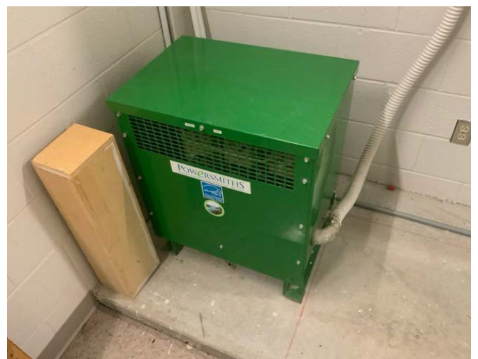
36 - SECONDARY TRANSFORMER
