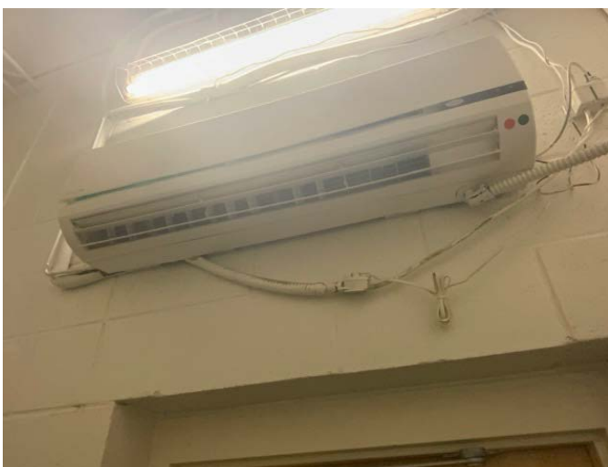
29 - INTERIOR SPLIT SYSTEM COMPONENT
