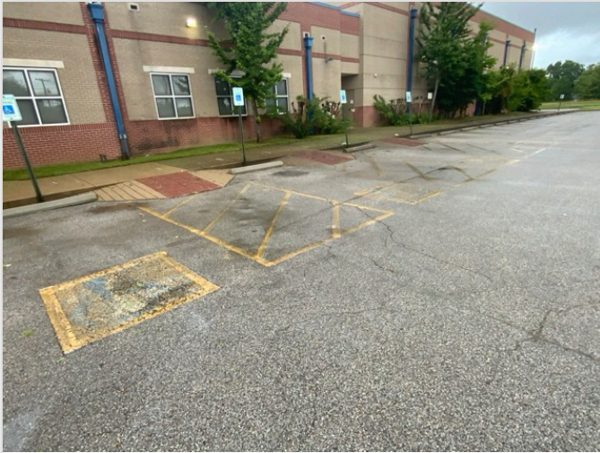
OVERVIEW OF ACCESSIBLE PARKING AREA
