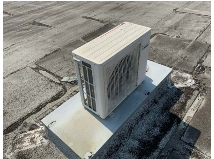
28 - SPLIT SYSTEM DUCTLESS
