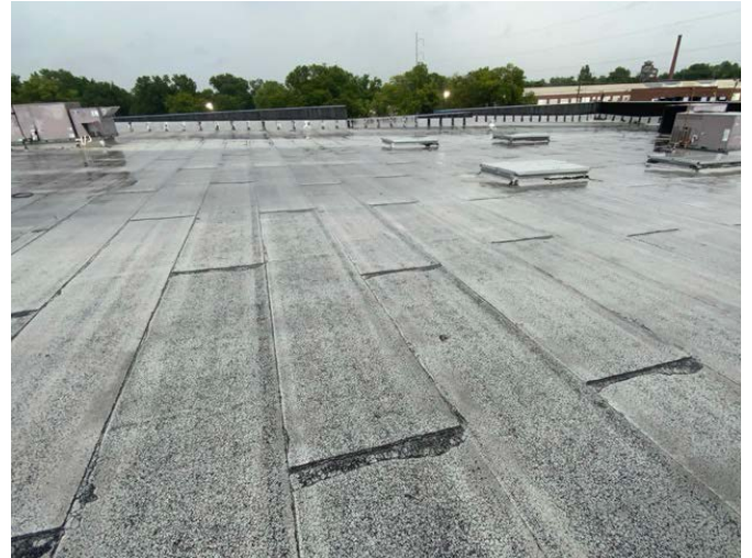
8 - MODIFIED BITUMINOUS ROOFING
