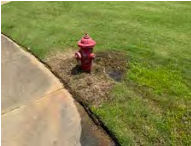
37 - HYDRANT (LEAKING)
