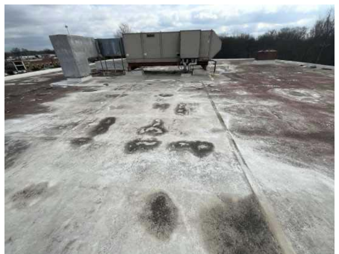
6 - TPO MEMBRANE ROOFING
