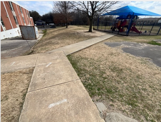
ACCESSIBLE ROUTE TO PLAYGROUND
