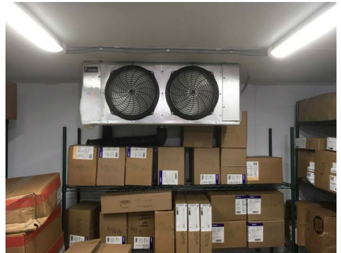
34 - EVAPORATOR FOR REFRIGERATOR/FREEZER
