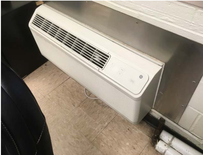
19 - PACKAGED TERMINAL AIR CONDITIONER
