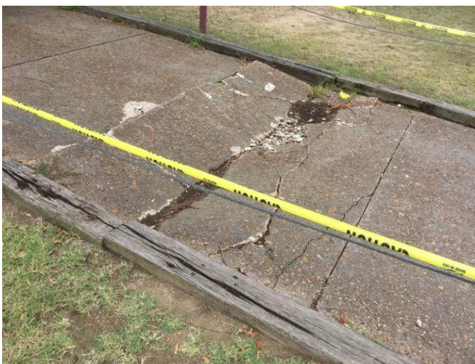
5 - CONCRETE SIDEWALK DAMAGE
