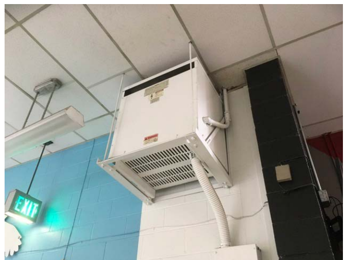
24 - SECONDARY TRANSFORMER
