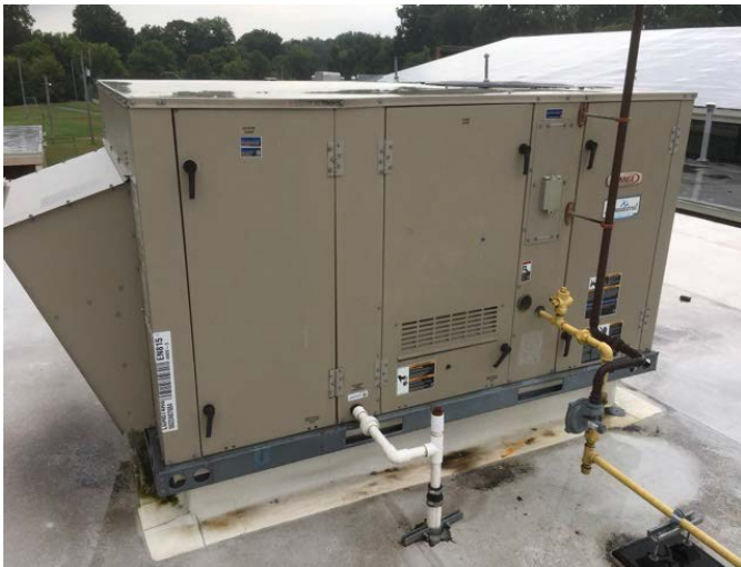
21 - PACKAGED UNIT, RTU
