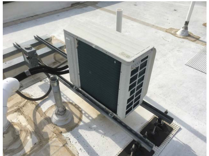
28 - SPLIT SYSTEM DUCTLESS
