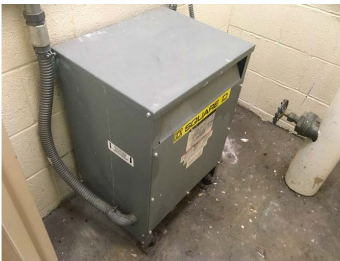
35 - SECONDARY TRANSFORMER
