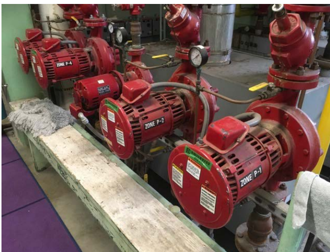
29 - PUMP, HVAC HEATING WATER
