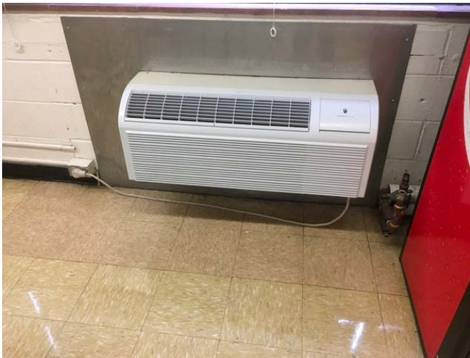
27 - PACKAGED TERMINAL AIR CONDITIONER
