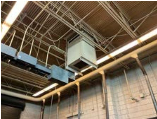
15 - BUS DUCT AND EXHAUST FAN
