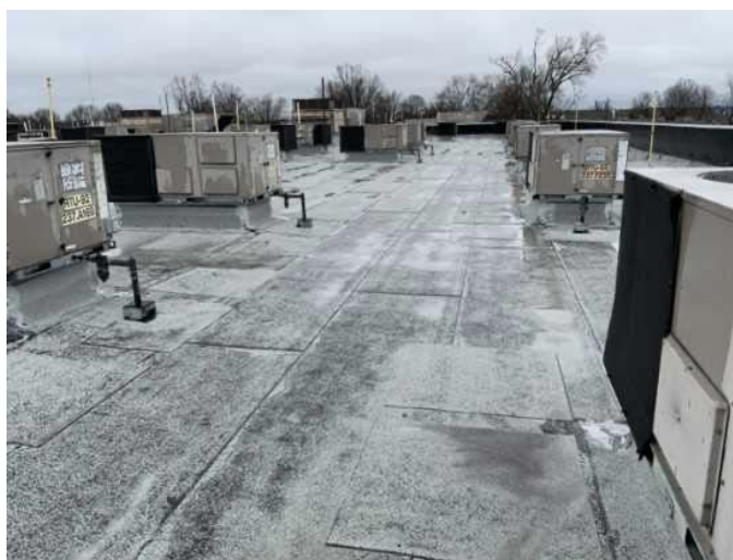
11 - PRIMARY ROOF OVERVIEW
