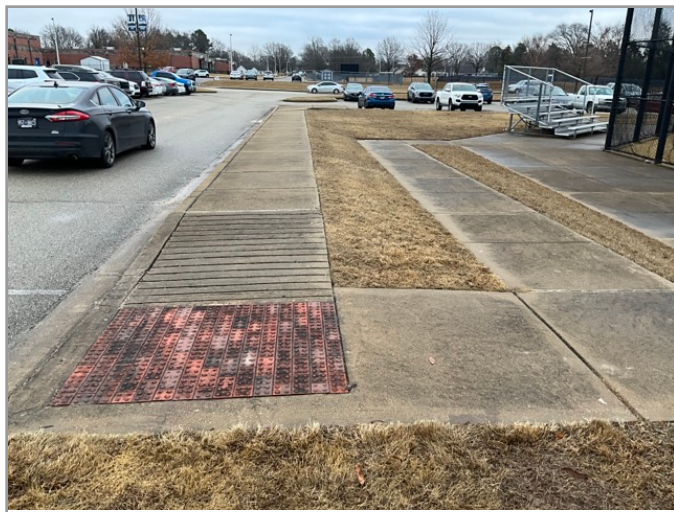
ACCESSIBLE ROUTE TO PLAYGROUND
