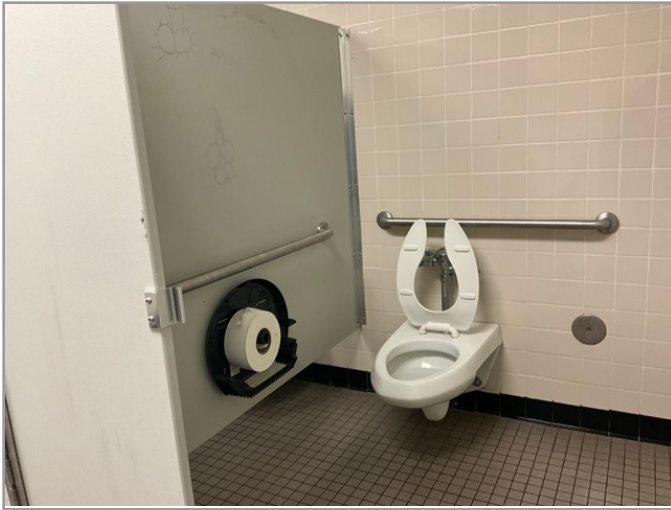
TOILET STALL OVERVIEW
