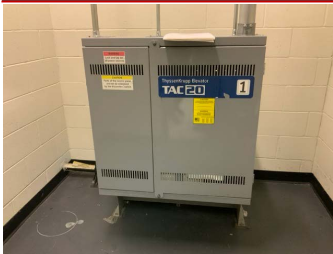
25 - ELEVATOR CONTROLS
