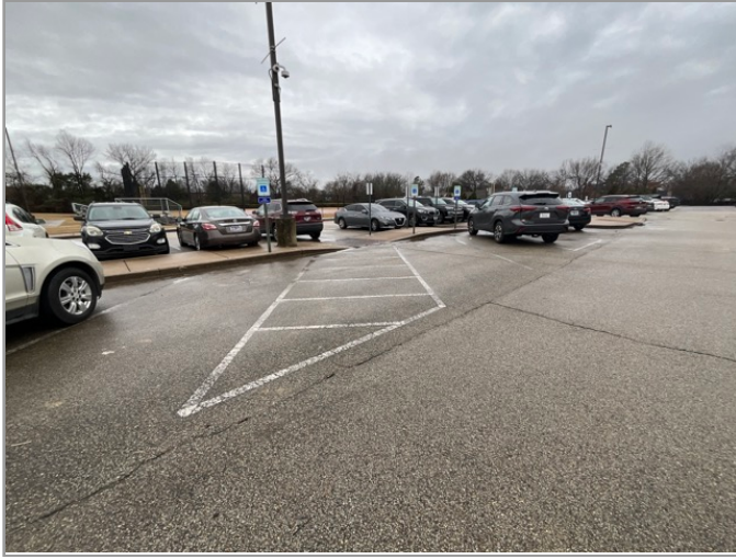
OVERVIEW OF ACCESSIBLE PARKING AREA
