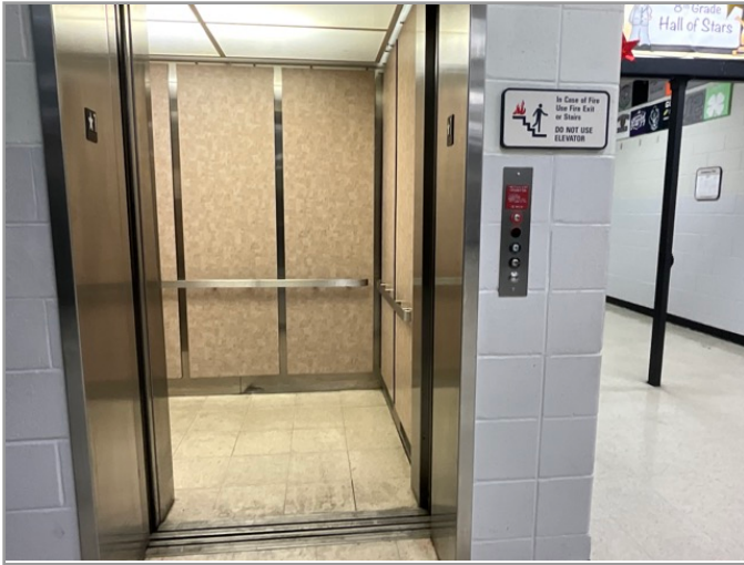
LOBBY LOOKING AT CABS
