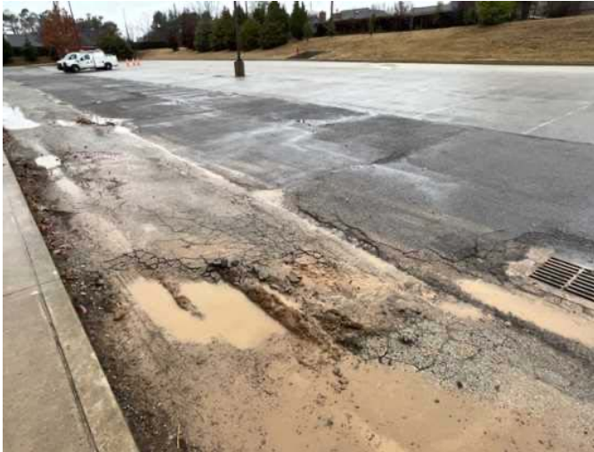
37 - SECONDARY PARKING AREA
