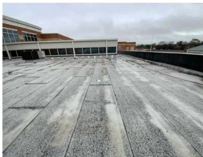
12 - SECONDARY ROOF OVERVIEW
