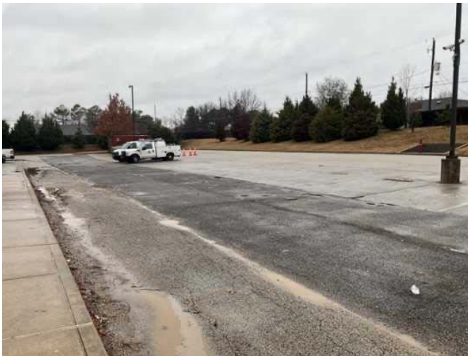
39 - SECONDARY PARKING AREA
