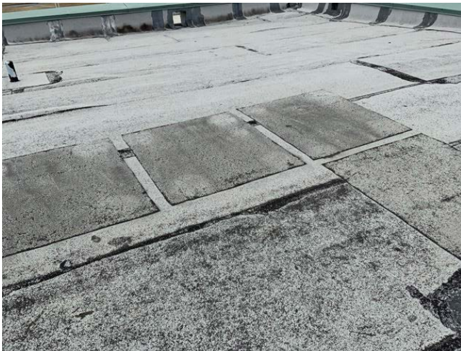
15 - ROOF OVERVIEW ANNEX
