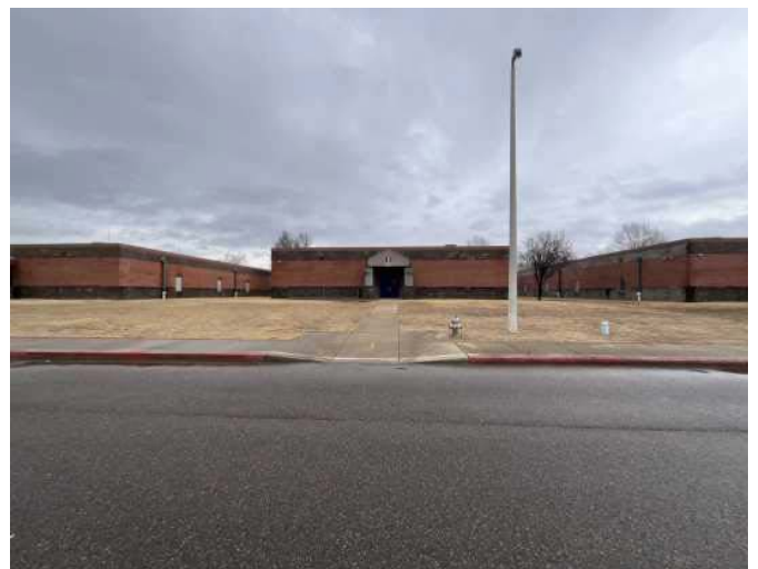
6 - LEFT EXTERIOR VIEW
