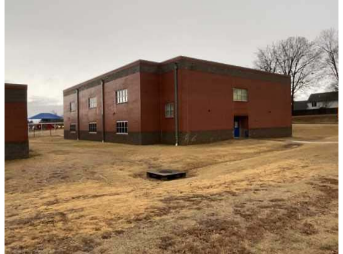
8 - RIGHT EXTERIOR VIEW ANNEX
