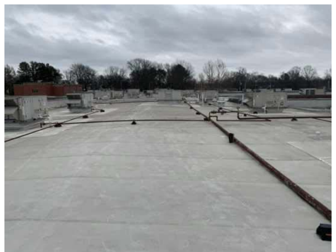
12 - PRIMARY ROOF OVERVIEW
