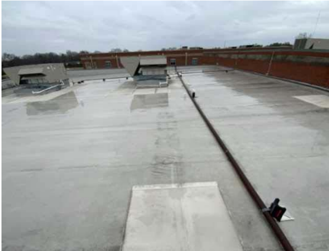
13 - SECONDARY ROOF OVERVIEW
