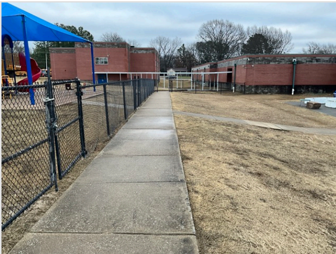
ACCESSIBLE ROUTE TO PLAYGROUND
