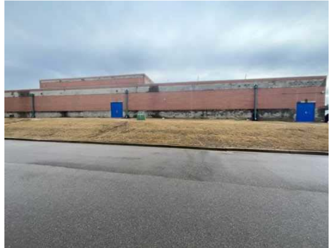
2 - RIGHT EXTERIOR VIEW
