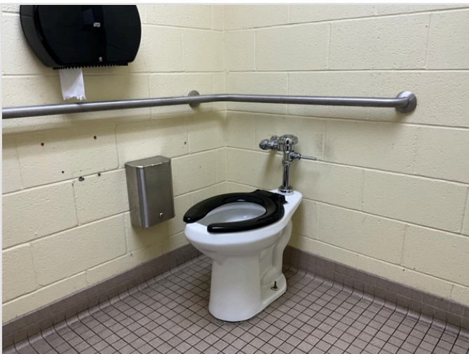
TOILET STALL OVERVIEW
