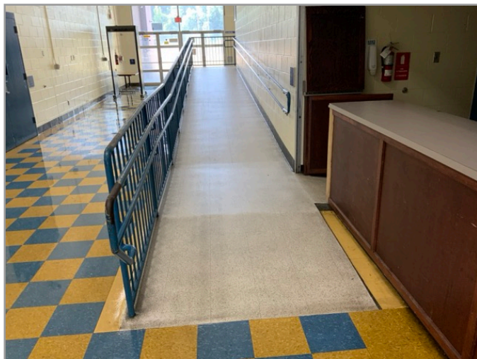
ACCESSIBLE INTERIOR RAMP
