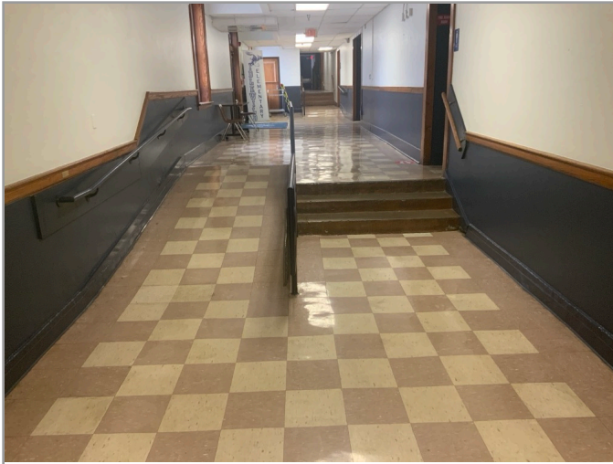
ACCESSIBLE INTERIOR RAMP
