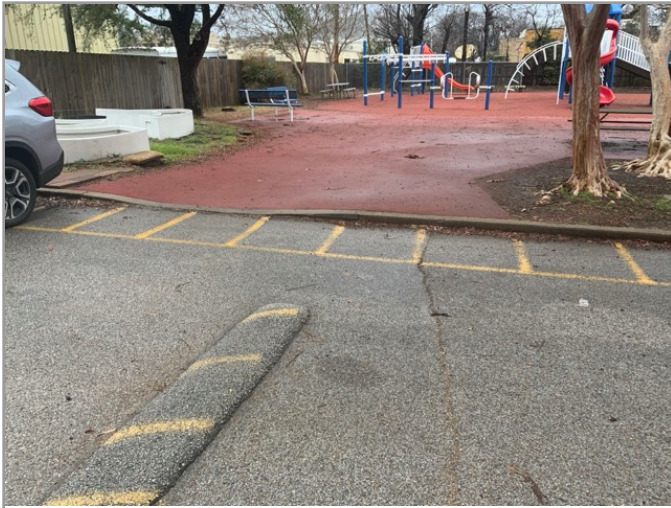
ACCESSIBLE ROUTE TO PLAYGROUND
