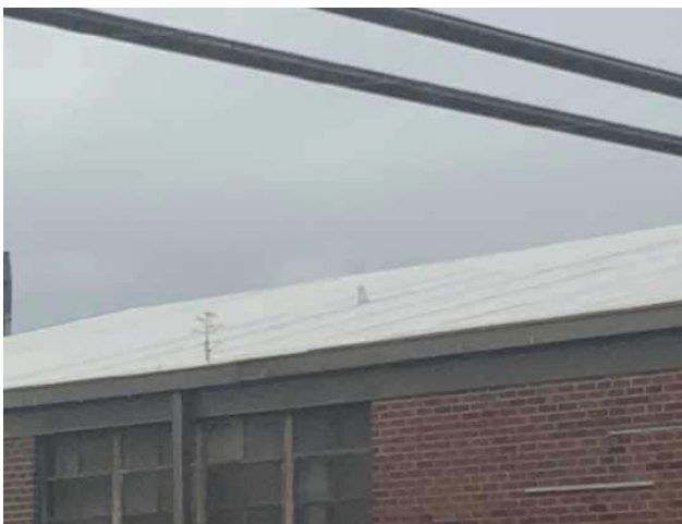
11 - ROOFING OVERVIEW - GYMNASIUM
