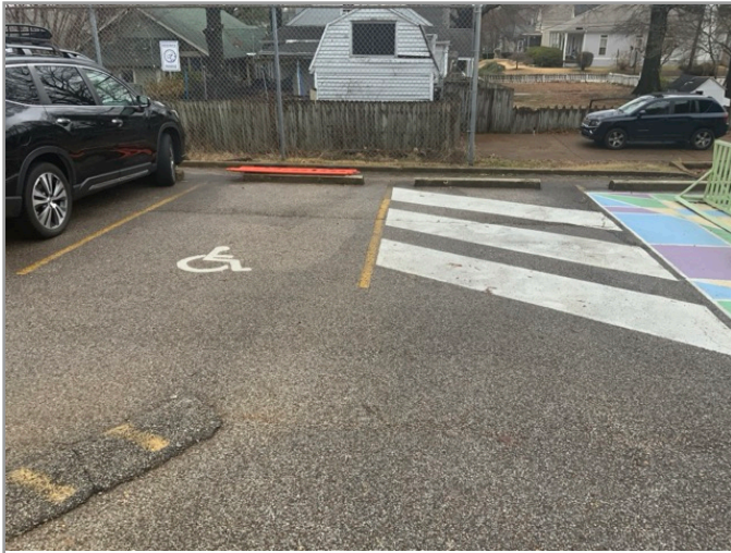
OVERVIEW OF ACCESSIBLE PARKING AREA
