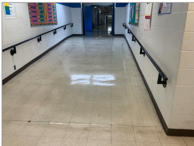
ACCESSIBLE INTERIOR RAMP
