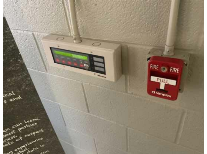
32 - FIRE ALARM SYSTEM COMPONENTS
