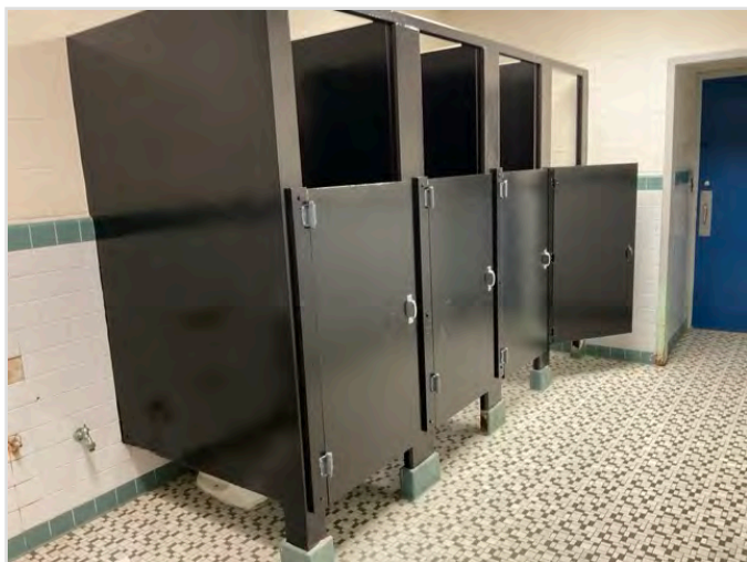
TOILET STALL OVERVIEW
