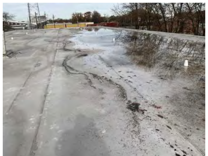
12 - MIDDLE SCHOOL ROOF
