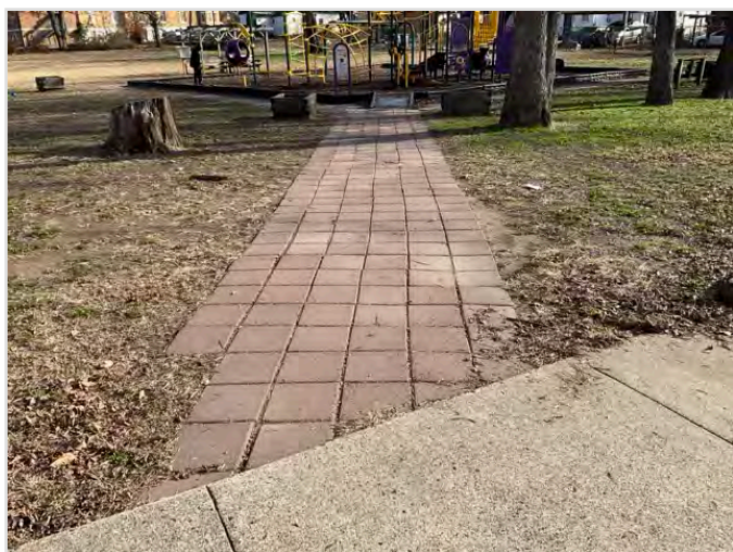
ACCESSIBLE ROUTE TO PLAYGROUND
