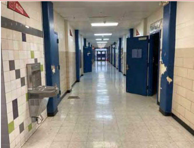
19 - MIDDLE SCHOOL HALLWAY
