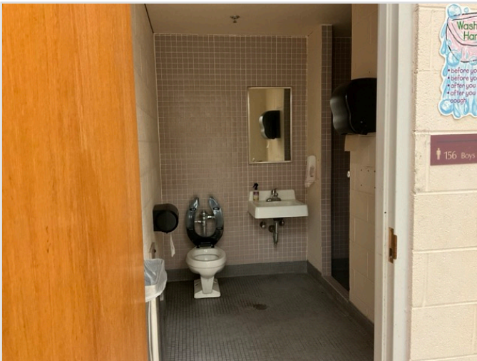
TOILET STALL OVERVIEW
