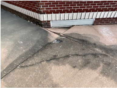
Sidewalk cracked at ramp - AssetCALC ID: 8455163
