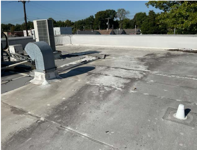
7 - ROOF (NEWER SECTION)
