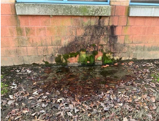
7 - DRAINAGE ISSUE AT FOUNDATION
