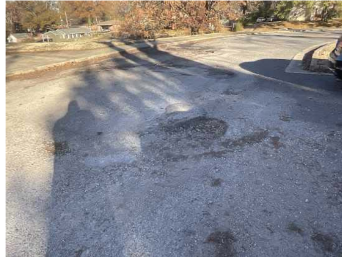
26 - ASPHALT POTHOLE
