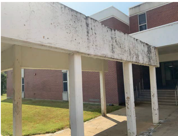
17 - FACADE MAIN CLASSROOM BUILDING
