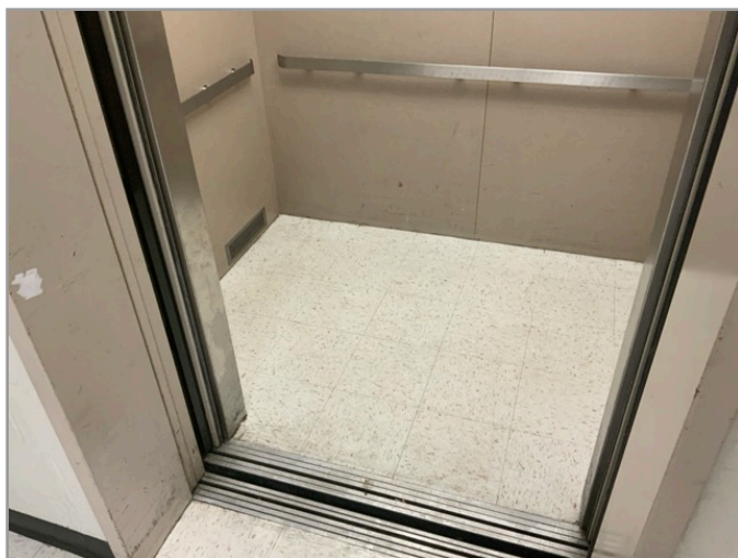
LOBBY LOOKING AT CABS (WITH DOORS OPEN)
