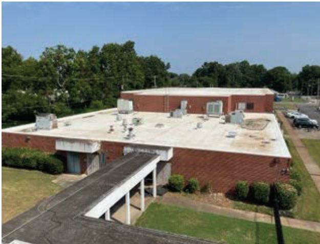
21 - ROOF OVERVIEW GYMNASIUM
