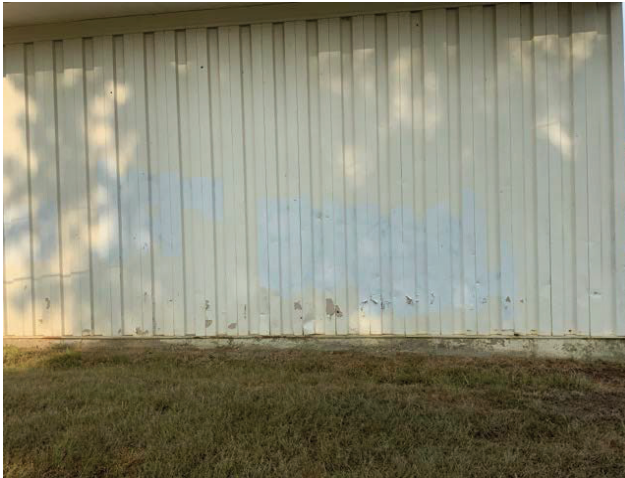
19 - FACADE AUTOMOTIVE SHOP
