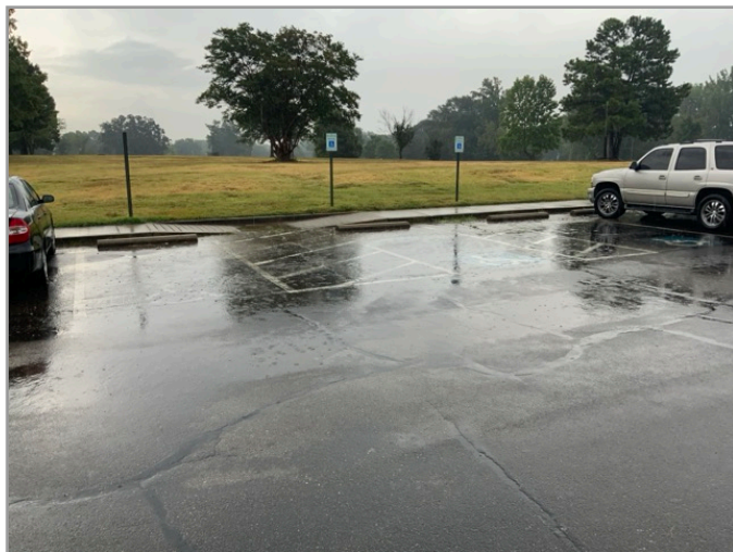
OVERVIEW OF ACCESSIBLE PARKING AREA
