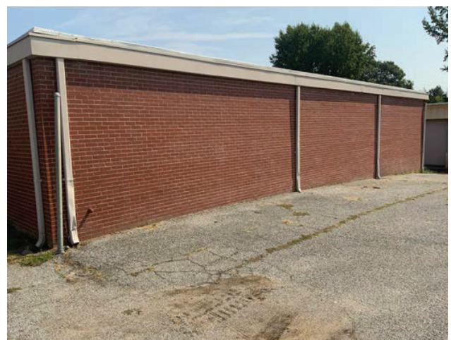
12 - RIGHT ELEVATION ROTC BUILDING
