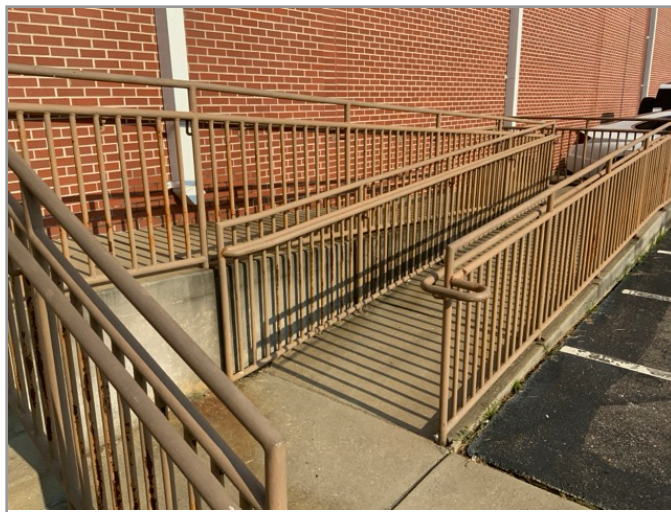
RAMP INTO BUILDING
